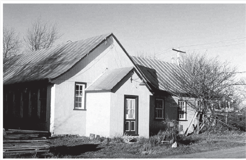
FIGURE 3 SCHOOLHOUSE, NEW GLASGOW, QUEBEC, BUILT IN THE 1840S
